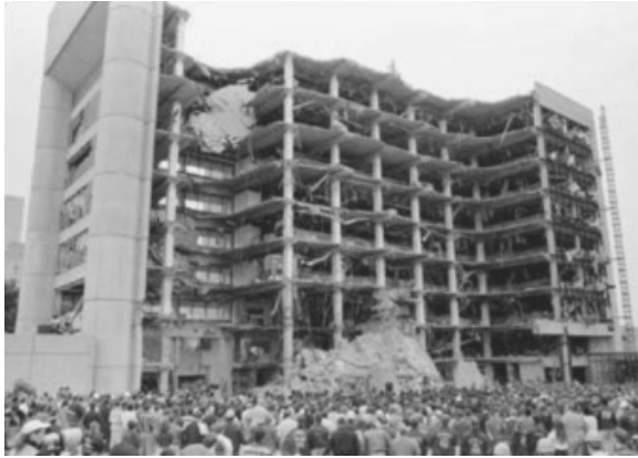
Figure 8.1 The Murrah Federal Building in Oklahoma City after the bombing in 1995.
